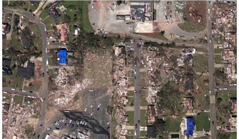
Tuscaloosa tornado damage (National Weather Service)
